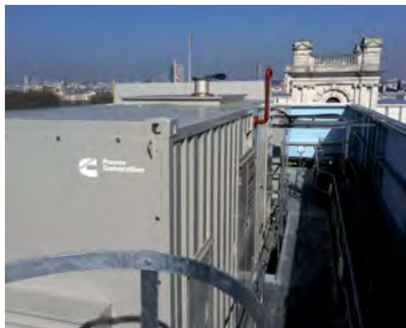
Cummins ESB installed a natural gas standby generator at the Institute of Civil Engineers in London.
