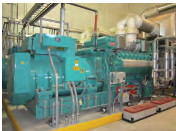
Two Cummins lean-burn natural gas generator sets provide standby power for Washington State University in the USA.
